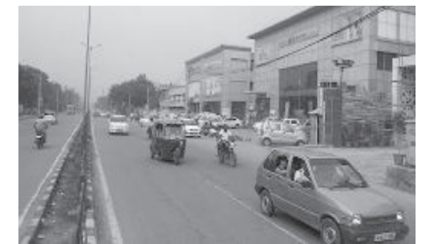
24 Metres Wide Road ROW Satguru Ram Singh Marg This road has the Green line Metro station called Satguru Ram Singh Metro station. This Metro station is 11 km from New Delhi Metro station.
