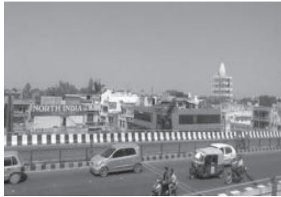
24 Metres Wide Road ROW Shivaji Marg Flyover Shivaji Marg Flyover is located in the Tihar sublocality of West Delhi.
